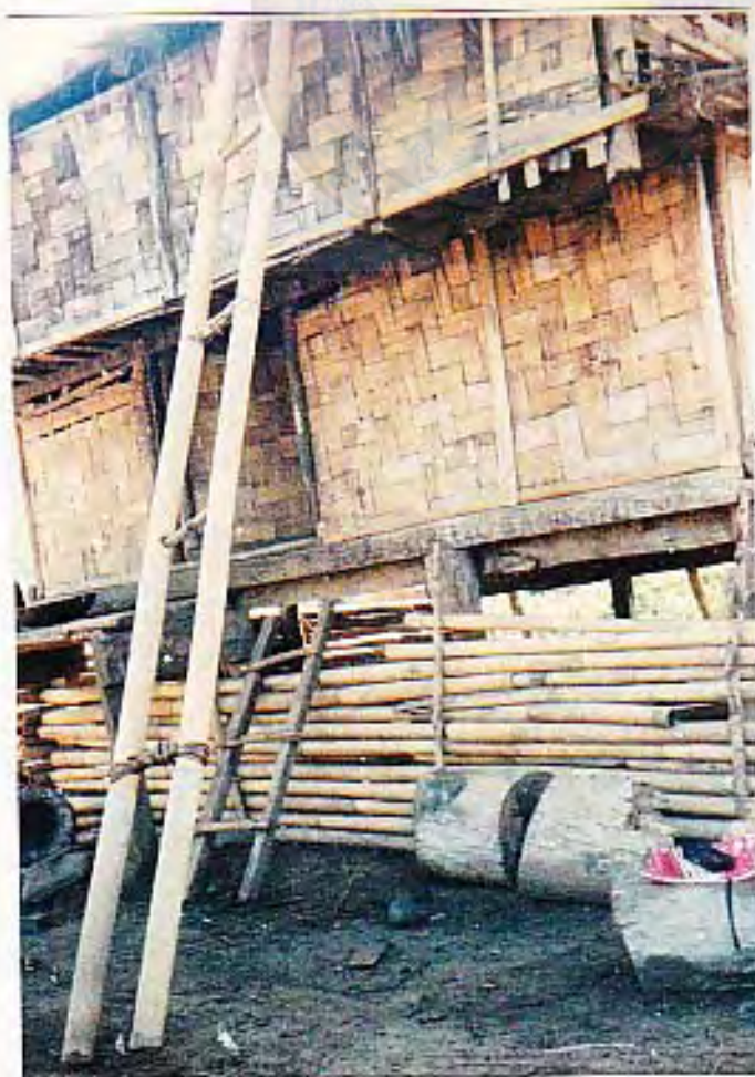
SAKLANG = Ladder out of bamboo
