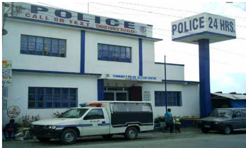
Plate 11. Municipal Police station of Buguias
