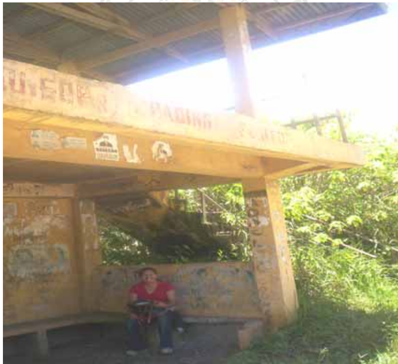
Plate 3. Waiting sheds; the lower plate shows a built-in loading platform on the second deck
