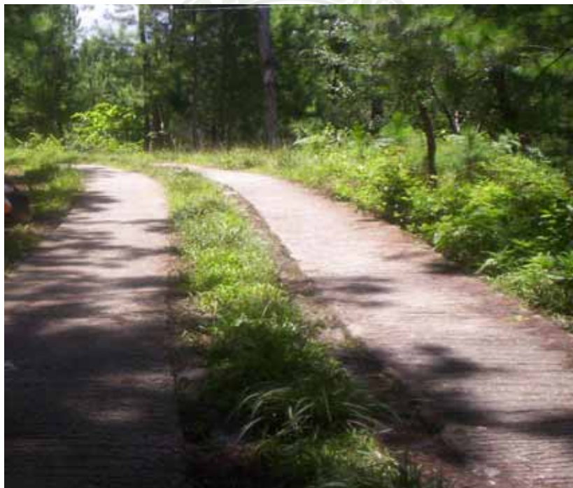
Plate 1. Portion of the community and farm road networks; upper plate shows a gravelled road and the lower plate shows that only tire paths are cemented
