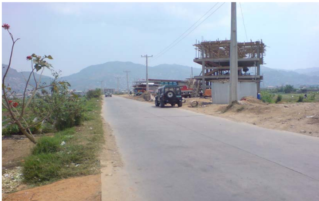
Plate 5. Concrete Road traversing Barangays Betag and Puguis (February 2010)
