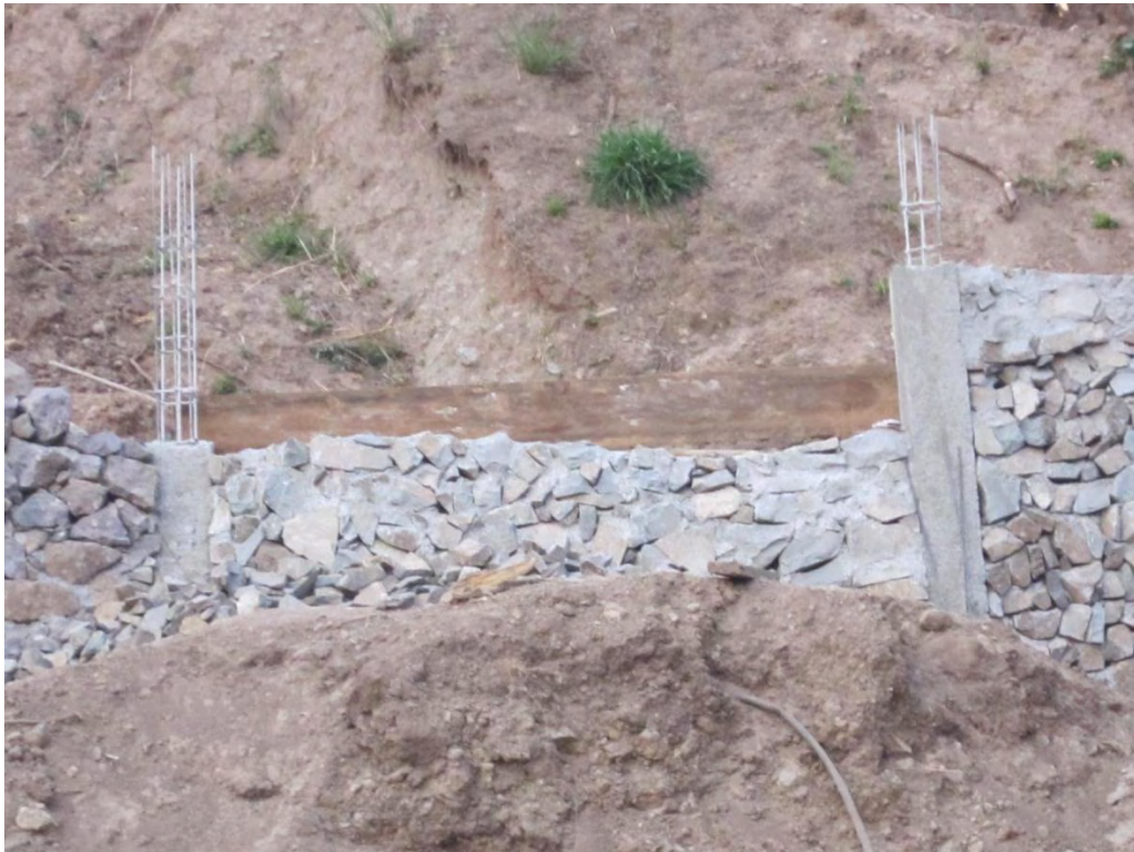
Plate 10. Riprapping of the field to prevent further erosion
