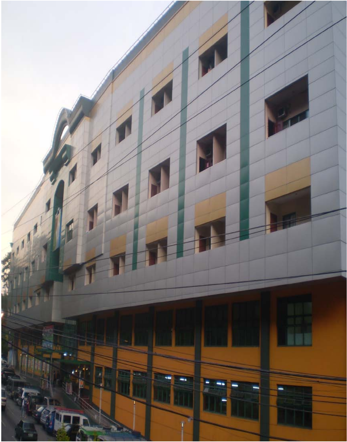
Figure 3. Building Structure of Cooyeesan Hotel Plaza, 2010
