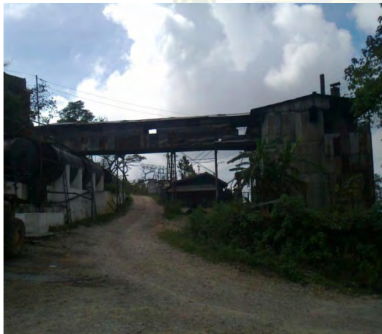
Plate 1. Lime Kiln Factory Photo by Amor Busacay, Dec. 2010
