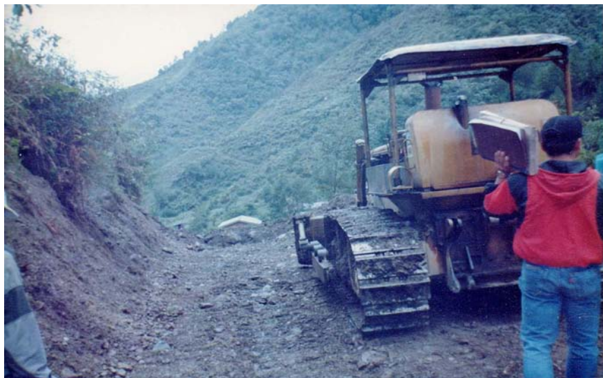
Plate 17. Tawangan Road Opening. CENRO Monitoring Report (1994)
