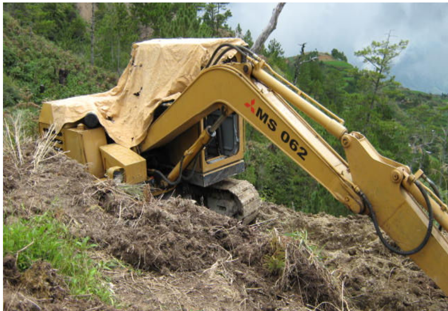
Plate 12. A backhoe parked, after clearing the forest in Tabeyo, Ballay. (August 25, 2009)
