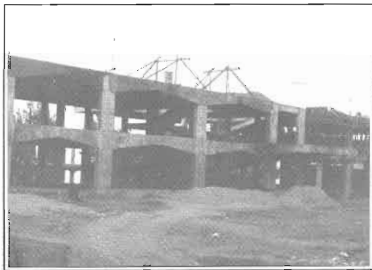
On-going construction of the College of Nursing building.
