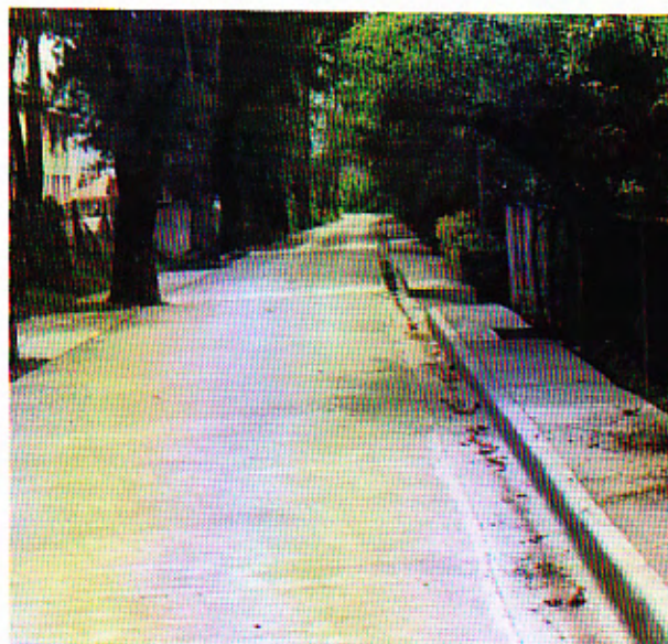
Road network constructed during the year at the staff housing
