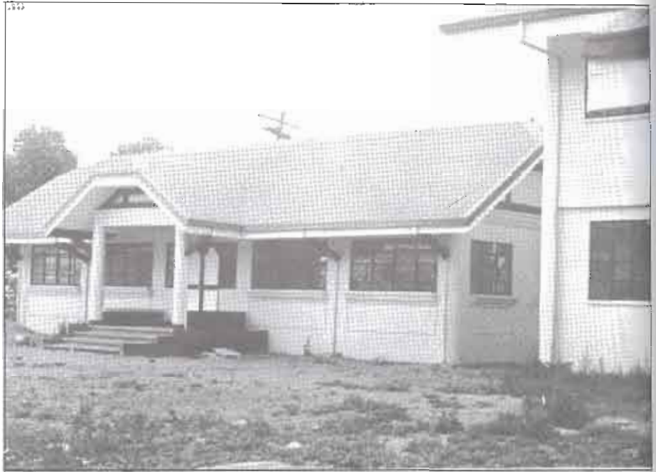
The BSU Teachers and Employees Association's Livelihood Center Building which was constructed out of the development fund given by former Senator Sotero Laurel to the association.
