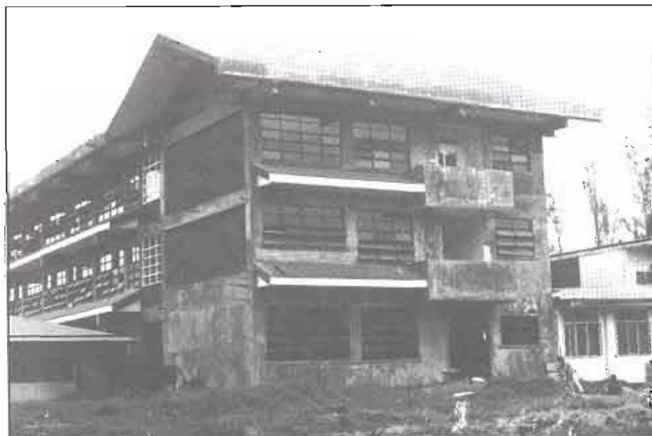
The College of Agriculture Building being constructed.
