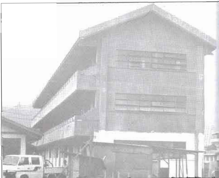
The College of Veterinary Medicine Building which is about to be completed.
