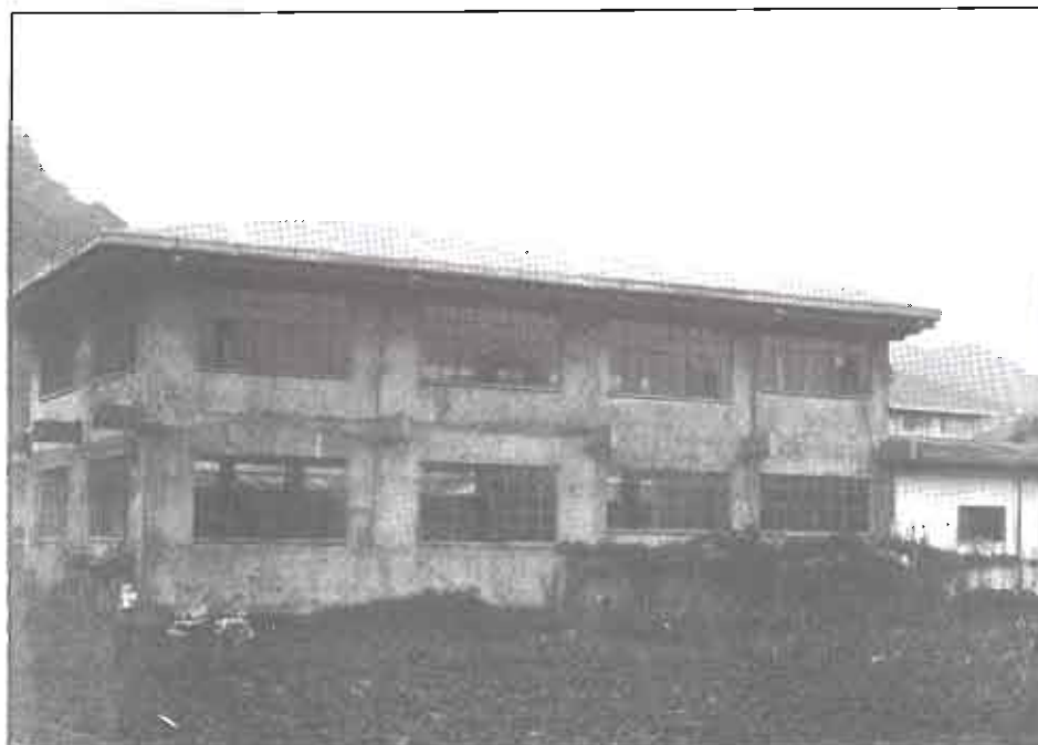
Extension Building of the Motor Pool to house Vocational Technology Fabrication Shop.
