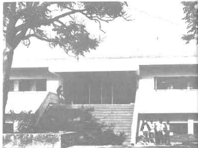
(Above) A portion of the damaged University Road is being repaired. (Lower) The University Library Building after it was rehabilitated from the damage wrought by the July 1990 earthquake. Other buildings and structures were likewise repaired with the release of P 25.6 million rehabilitation fund for the university.
