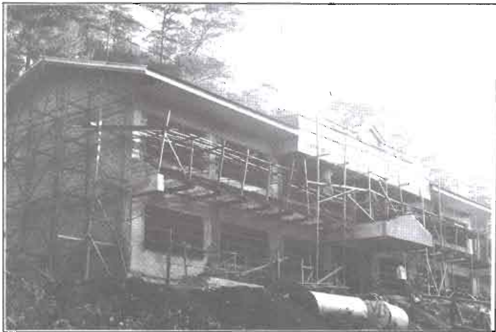
On-going construction of the College of Forestry
