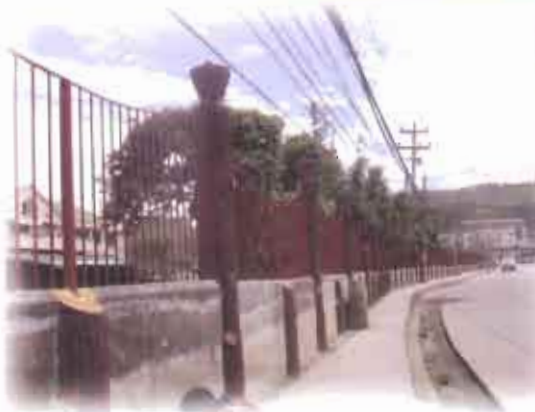
Completed fence at Km 5
