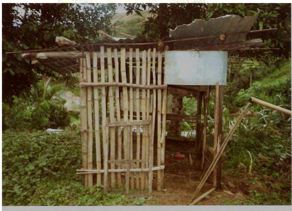
Figure 15. The shed-type of housing in Kasibu, Nueva Vizcaya
