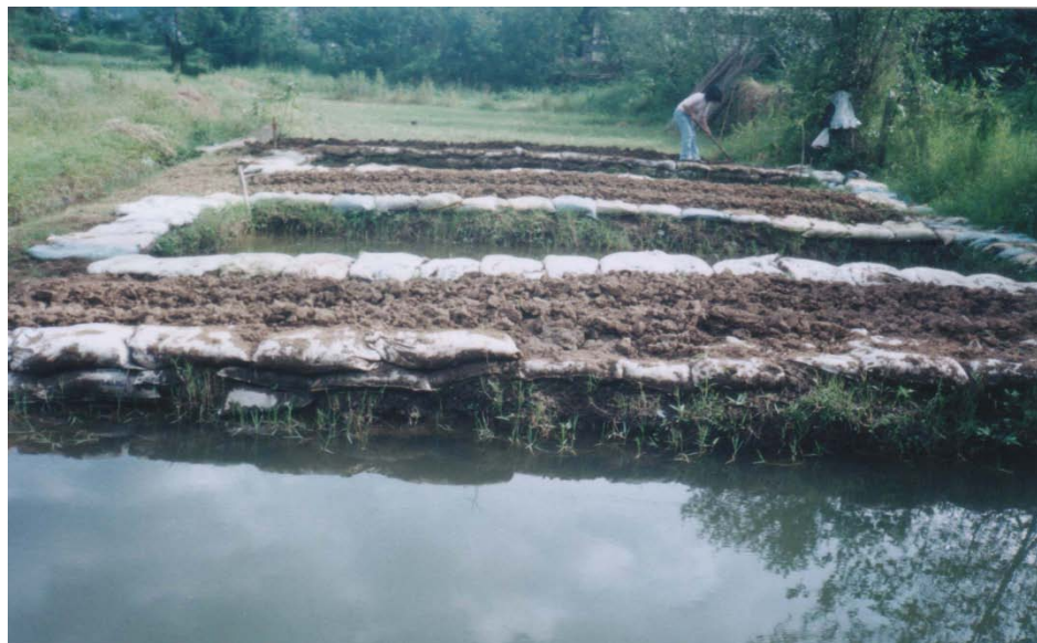
Plate 1. The newly established system showing the dikes stabilized by sacks
