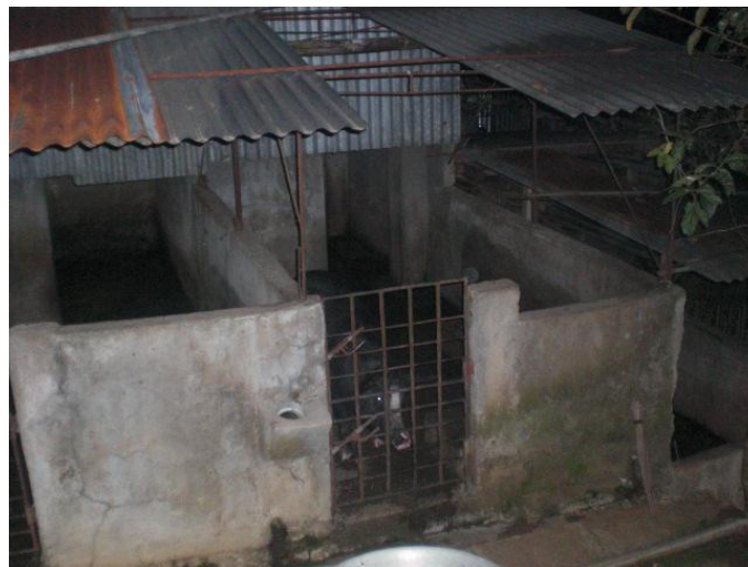
Figure 12. GI roofing with solid concrete walling and flooring
