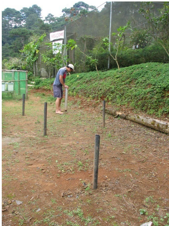
Figure 14. Installation of the plastic pipes
