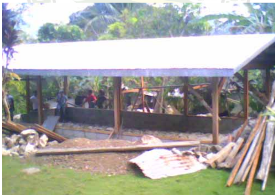
Figure 3. Semi-concrete rearing house
