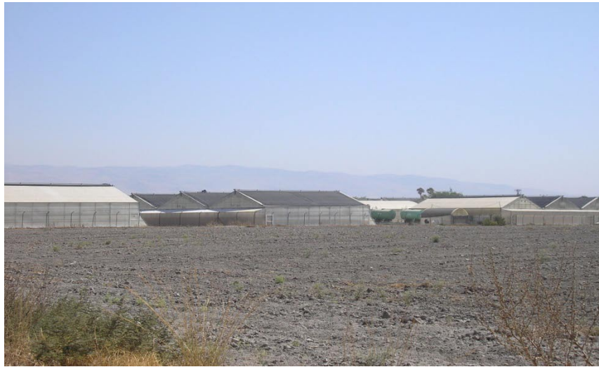
Figure 2. Greenhouses in Beit Shean Valley
