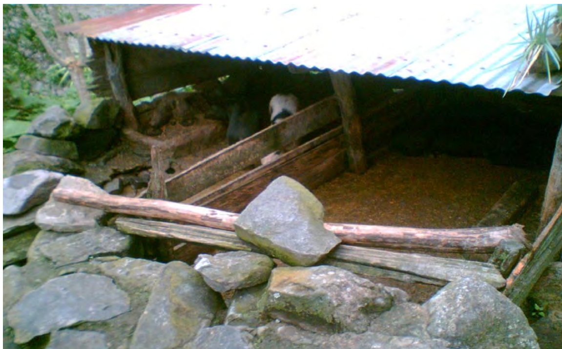
Figure 3. A swine house with stone walls and galvanized roof owned by one of the respondents in barangay Gawana (pob)
