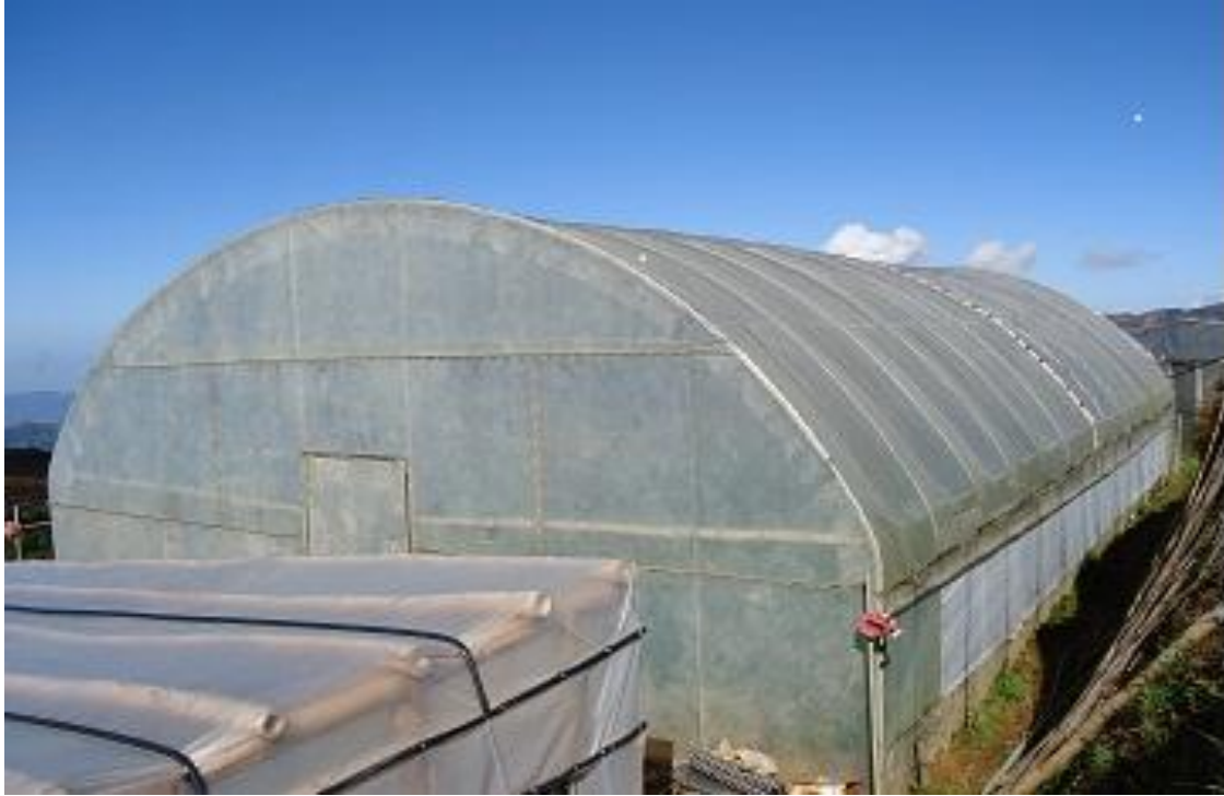
Figure 1. Overview of the tunnel type greenhouse at Atok, Benguet
