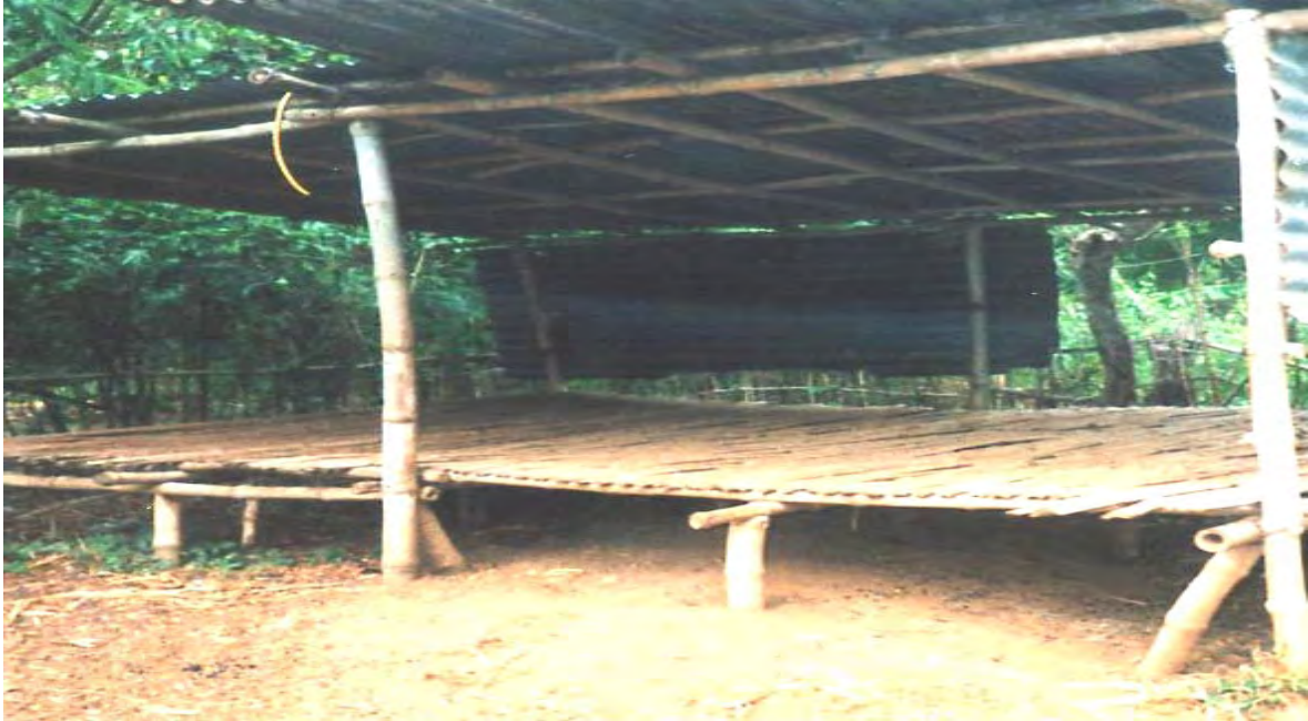
Figure 24. Elevated housing of goats made of bamboo flooring and G.I. sheets roofing
