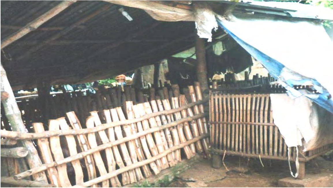
Figure 11. Swine housing with bamboo walls and a brooder beside the house
